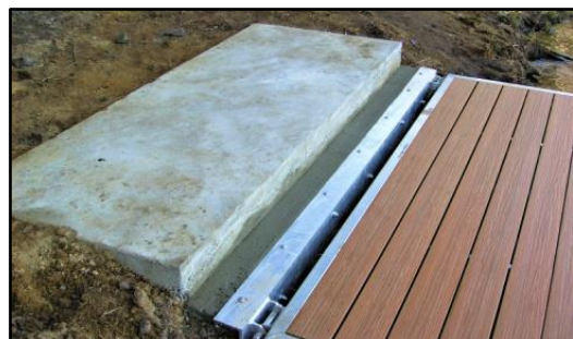
Concrete Angle on New Concrete
